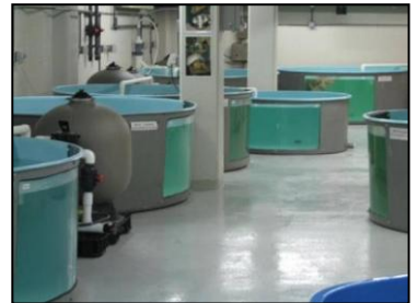
Indoor facility, note windows built into the tanks for viewing, © B. Bergwerf, SCA
