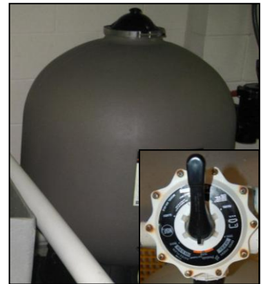
Sand filter, © J. Bluvias Insert: Multi-port valve, © S. May, NCA-PKS
